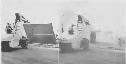
LIRE A dentist pulling teeth, this specialized vehicle jerks out storage tank sections with speed and ease. The steel sections are slated for the scrap pile.
